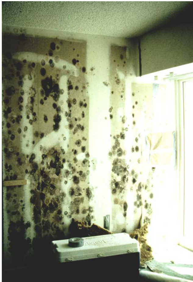
Photograph 2: Vinyl wall covering removed to expose mold on hotel room wall
